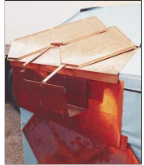
Mock-up of the tiles, gutter and strapping, and copper fascia assembly.
