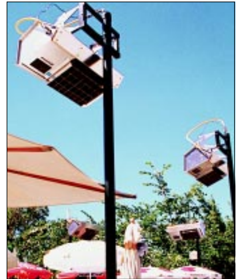
Each infrared heater can heat an area of 110 to 160 sq. ft. (10-15m 2 ).
