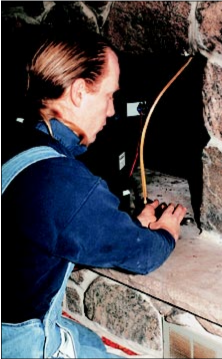
Bill Watt of Gowing Gas Plus connecting a copper supply line to the fireplace insert for the Owen Sound residence.
