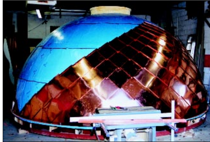
The Holy Family Church dome during shop fabrication.
