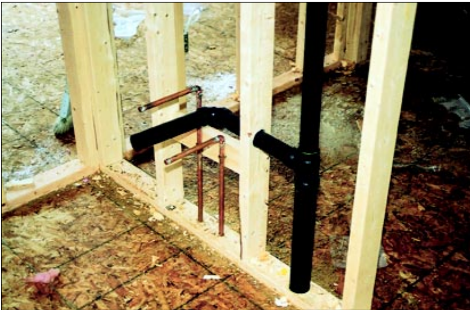
Type M copper tube is used for hot and cold water lines in Sunvale Homes.
