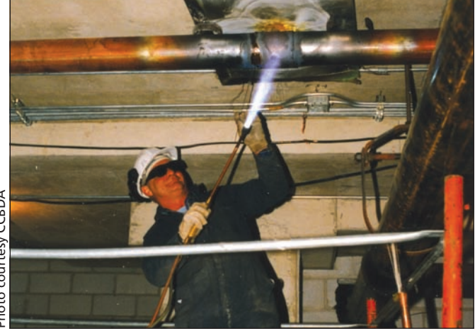
Brazing a 5-inch Type K copper vacuum line in a hospital.
