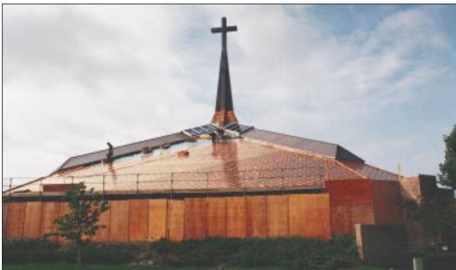
St. Justin's Church, with the newly installed flat seam spire and CastleTop Metal Tile roof.
