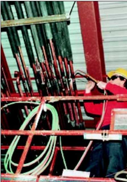
Brazing overhead lines of hard drawn copper tube.
