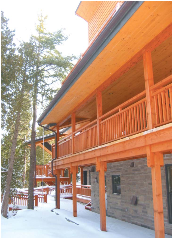
The building exterior also features copper gutters, vents, and hardware.
